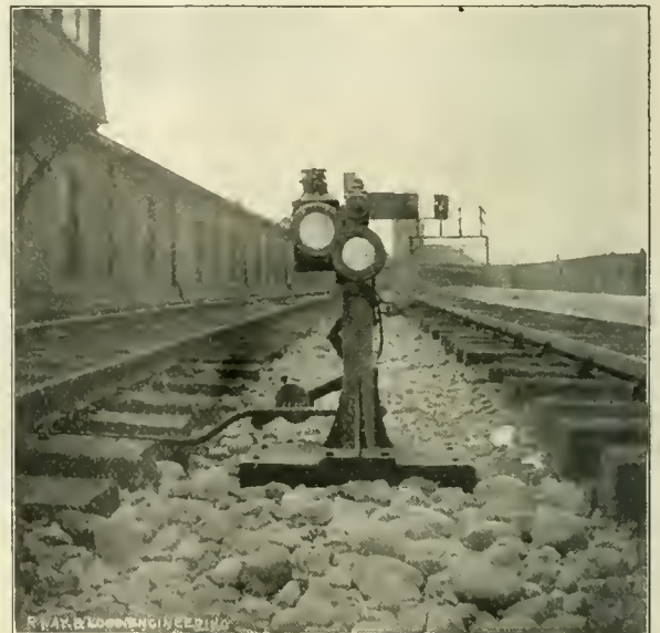
DWARF SIGNAL, USED IN BACKING UP MOVEMENTS.
